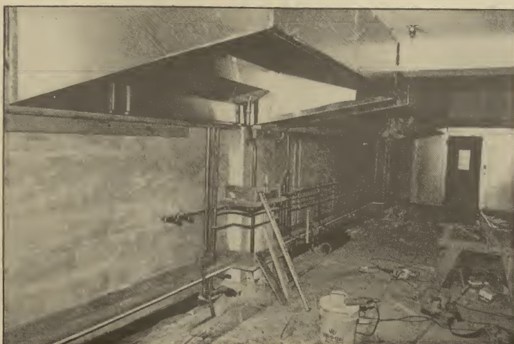
The new kitchen goes in at Project Open Hand.
